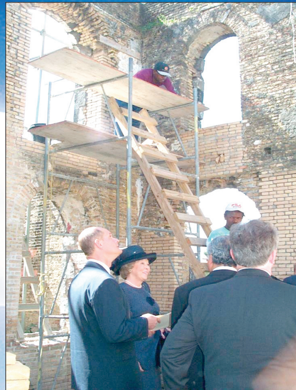
Queen Beatrix of the Netherlands visited the Honen Dalim synagogue in St. Eustatius in January 2001. The Queen visited the synagogue, when it was still under renovation, as part of a walk through the Historic Chore. Photo by Suzanne Koelega.
